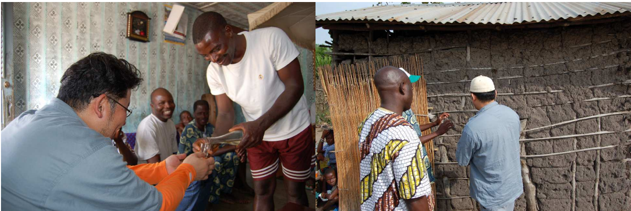
(Left) at the village chief house in Kpetou, welcome ceremony with slabi , the strong spirit (Right) Kpetou is located inland in comparison with Possotome, thus the clay is less viscous and sandy, easily fissured and needs wooden reinforcements
