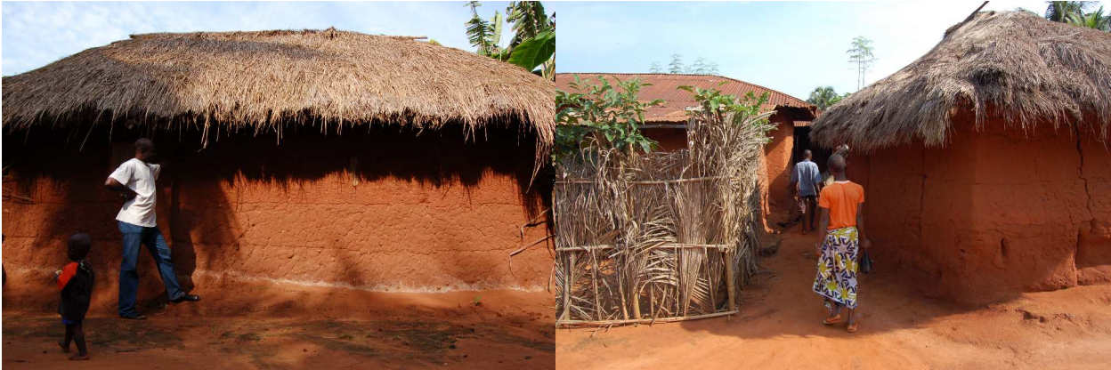
(Left) traditional house in Possotome: blocks are piled up about every 50cm, takes 2 weeks to dry, construction period can be calculated by the total number of blocks (Right) local guide takes the back streets of Possotome, an interview site
