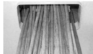
Remove oil sludge, etc. from coamings before putting cables together.
