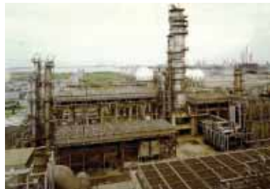
Heat transfer technology (Air-cooled heat exchanger for petrochemical plant)
