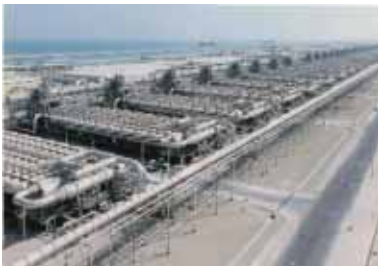
Water treatment technology (Desalination Plant for Middle East)
