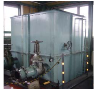
LUB. OIL PUMP TEST SHOP
