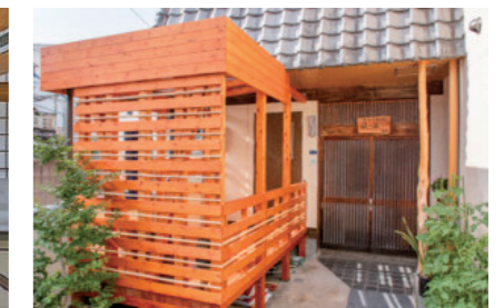
A house located facing the old highway along with traditional houses. The house is renovated, utilizing the small courtyard, and adding a wooden deck. (Kaze-no-Siori, Osaka City)
