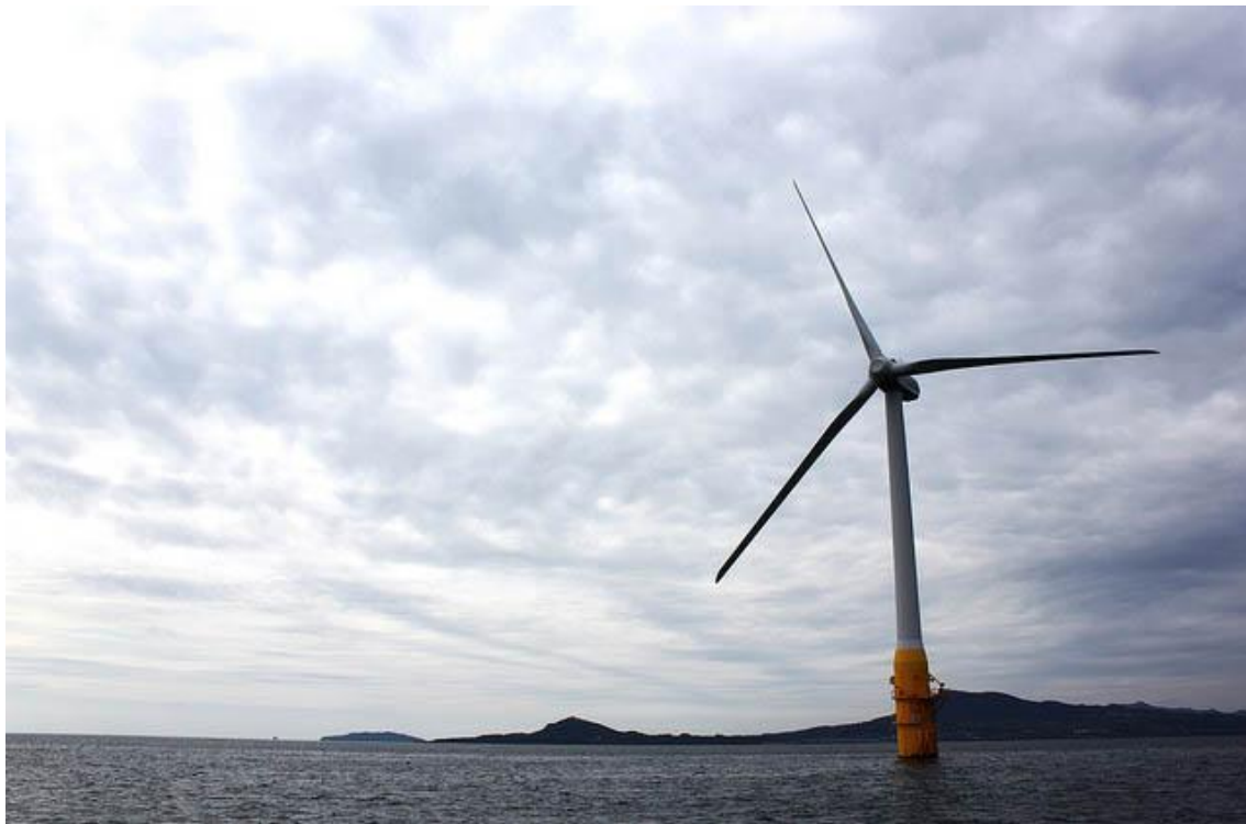
五島の洋上風力発電の構造体 Goto Floating Offshore Wind Turbine (Sakiyama) photo by mmatsuura Follow(frickr)
