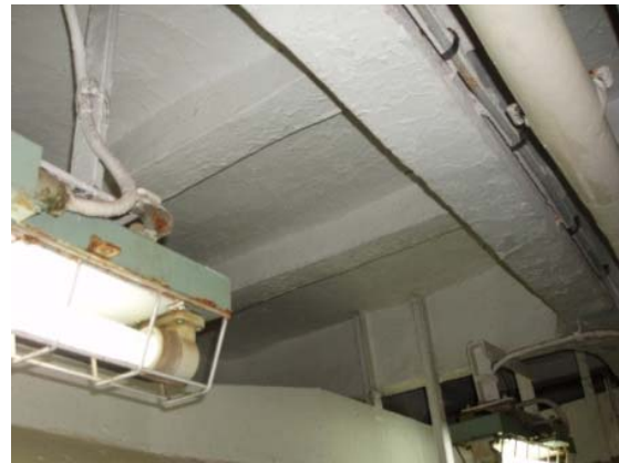
(Asbestos sprayed on ceiling to prevent dew condensation)
