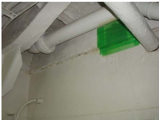
(Sprayed-on surface is held in place by plaster. The right photo shows a section in which part of the surface has been removed.)
