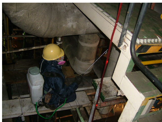
(Moisturizing asbestos using atomizer)
