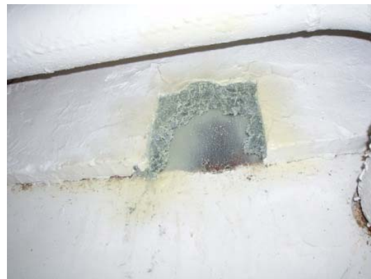
(Sprayed-on surface is held in place by plaster. The right photo shows a section in which part of the surface has been removed.)
