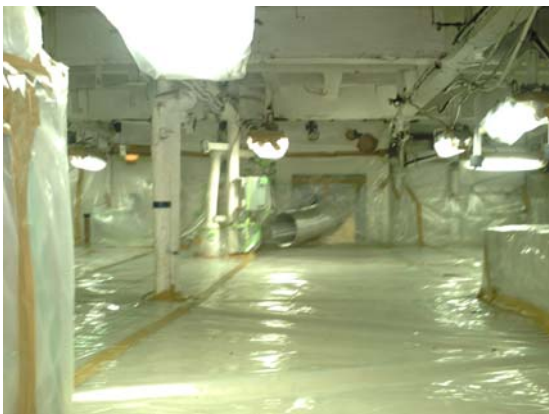
(Two polyethylene film sheets; duct leading to negative-pressure dust collector)
