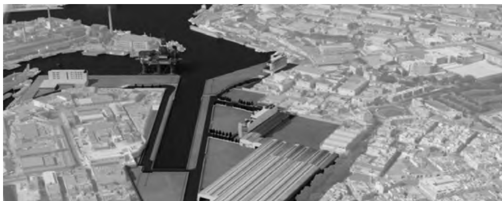
Figure 5: The facilities of the Mediterranean Maritime Hub as they are being redeveloped. (Source: MMH).
