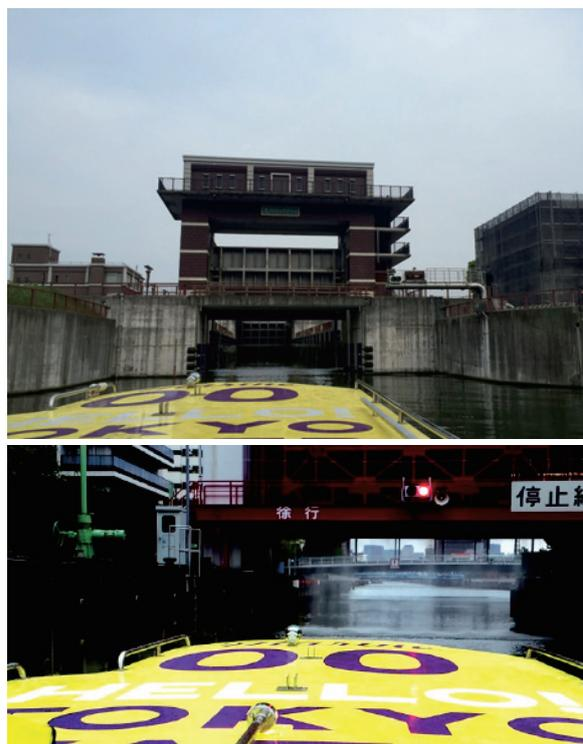
The gate closes after you enter from the river. Then, water is drained out and the water level is lowered below that of the river. When the water is at the correct level, the sluice on the opposite side opens, and you can advance into the canal. When going out of the canal, the opposite procedure is performed.
