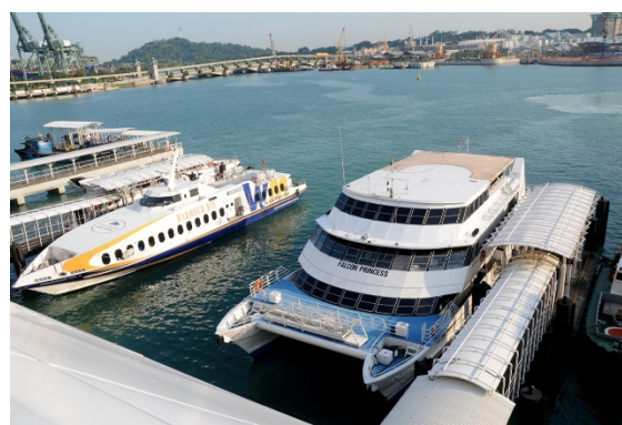
Regional Ferry Terminal (RFT)
