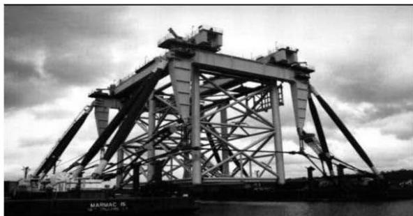
Versatruss Jacket Lifting System Topside/Jacket Lifting
