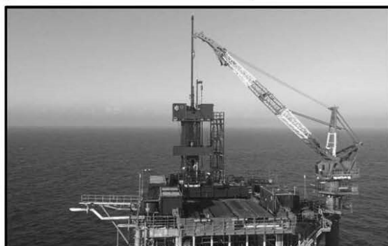
Hydraulic Workover Unit (坑井介入作業)
