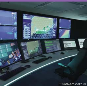
Fleet Support System Console
