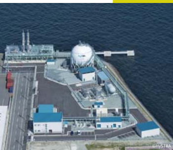
Liquefied Hydrogen Terminal 'Hy touch Kobe'
