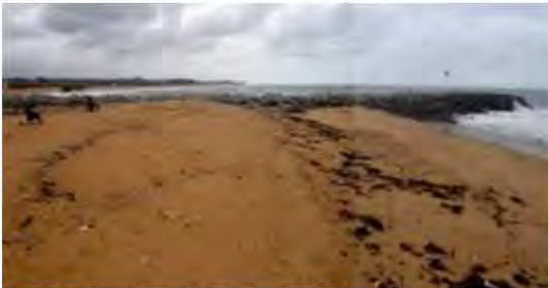
Photo 4: Cove formed by erosion downstream of the 2014 groin field
