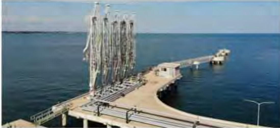
Photo 16: Second hydrocarbon station
