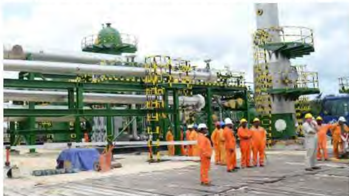
Oil and gas facility in the Niger Delta
