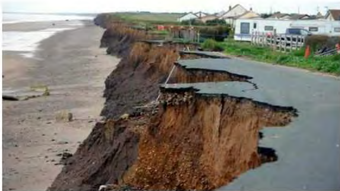
Coastal erosion along the coast of Bayelsa state, Nigeria
