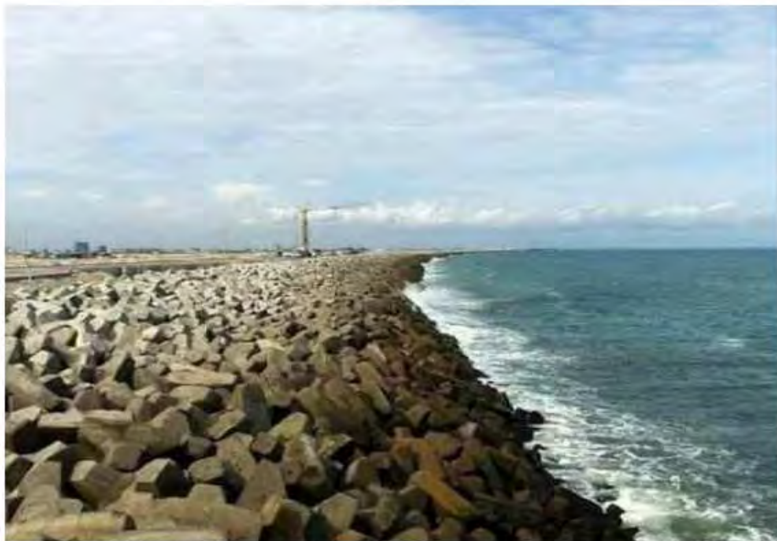
Coastal defense infrastructure by Lagos state government
