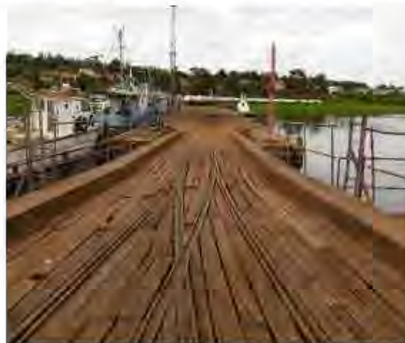
Link span at Port Jinja
