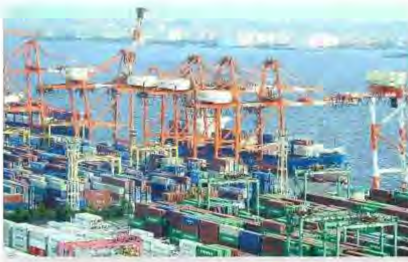
Container yard in Tokyo - Photo by Ari Ara on Unsplash
