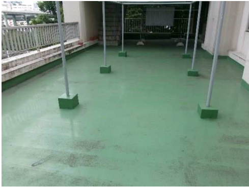
(2階屋上陸屋根) 床防水打ち替え
