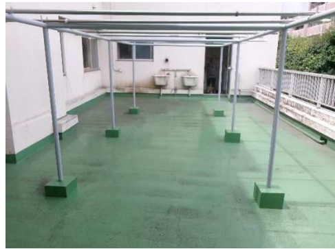
(2階屋上陸屋根) 床防水打ち替え
