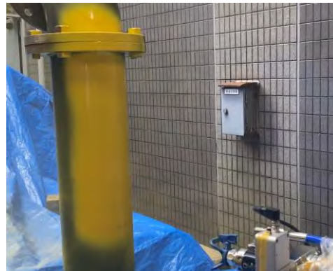
First attempt in pipe painting (pressure: 1000 psi, distance 12in, robot speed 60%)
