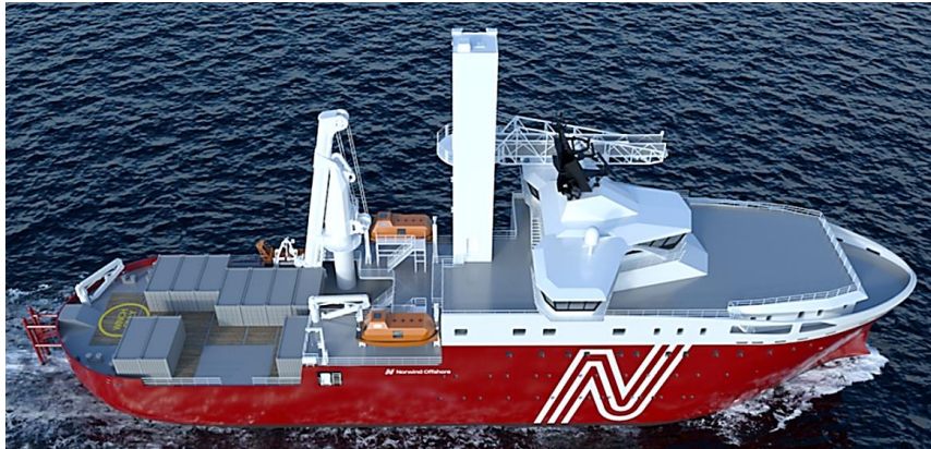
図 25 Vard 419 CSOV under Construction in Vietnam
