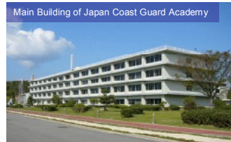
Main Building of Japan Coast Guard Academy
