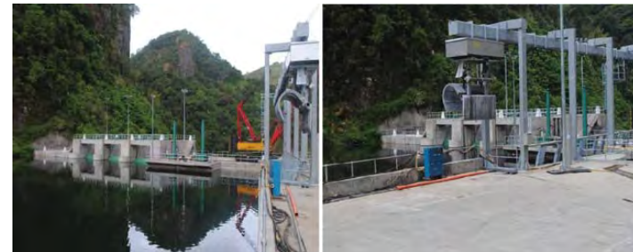
Nadarivatu Hydro-Electric Power Project, Fiji
